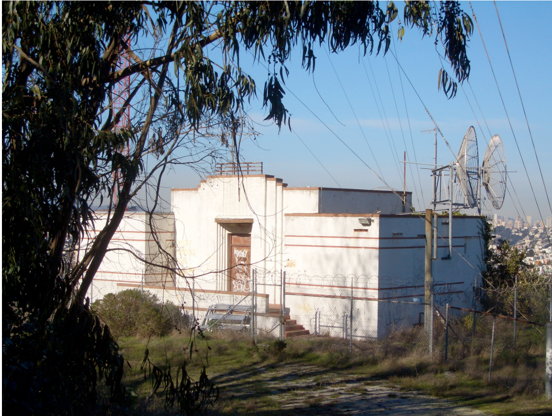
Julia Morgan Designed Transmitter Site. Built in 1937.
